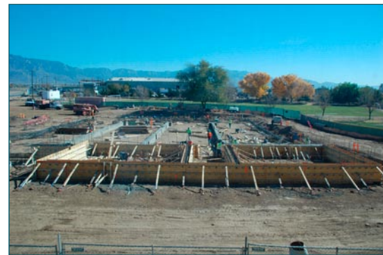
Sandia Prep's new Field House on Nov. 27, 2007
