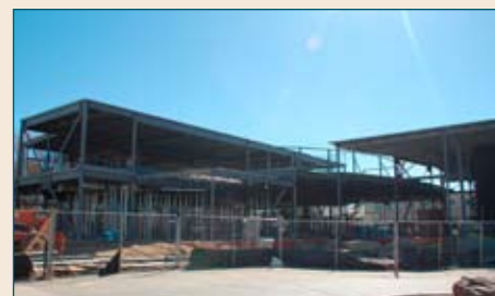
SPS Performing Arts Center from the northwest, 2.3.09
